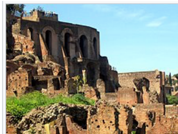
Massive retaining walls extended the area on the Palatine available for the Imperial building complex.
