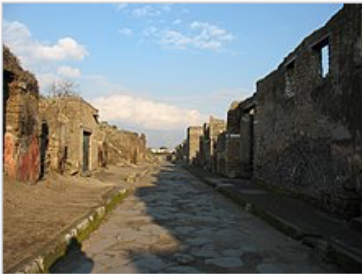
The buildings on the left show signs of decay due to the infestation of various plants, while the debris accumulating on the footpath indicates erosion of the infrastructure. The footpaths and road have also been worn down by pedestrian activity since excavation.
